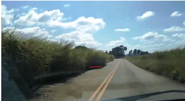
Figure 3. Section of LMG-878 with lack of maintenance regarding the roadside vegetation. The red line is 1.5 m towards the center of the carriageway.
